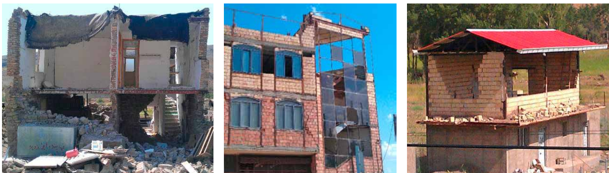
Fig. 2. An example of earthquake area destruction due to seismic loads
