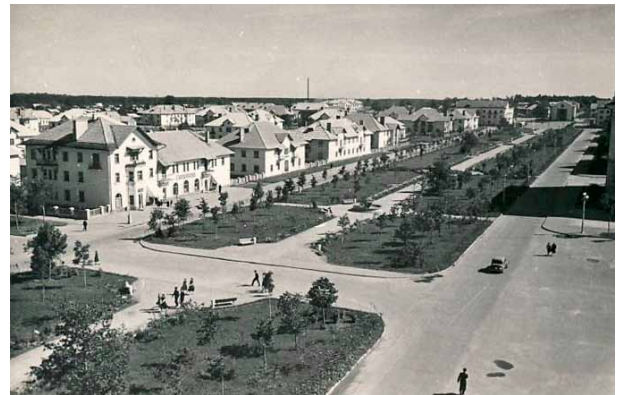
Fig. 11. Stalinist centre of Kohtla-Järve, early 1950s by Lengorstroyproyekt. Photo taken in 1950s (RM F 646.176)
