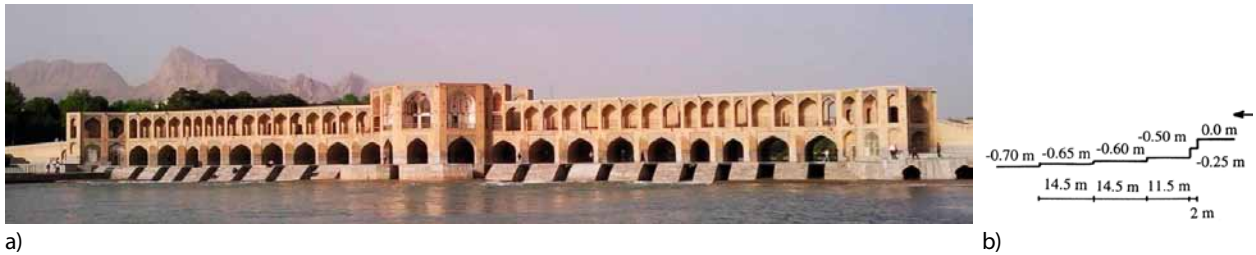
Fig. 30. (a) The Khaju bridge; (b) the bed slope of a canal intake, Isfahan, 1650 A.D.
