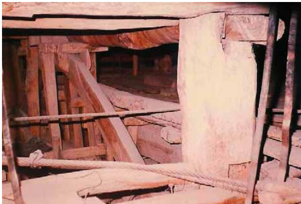
Fig. 28. A wooden truss, Ali Qapu building, Isfahan, 1597–1668 A.D.
