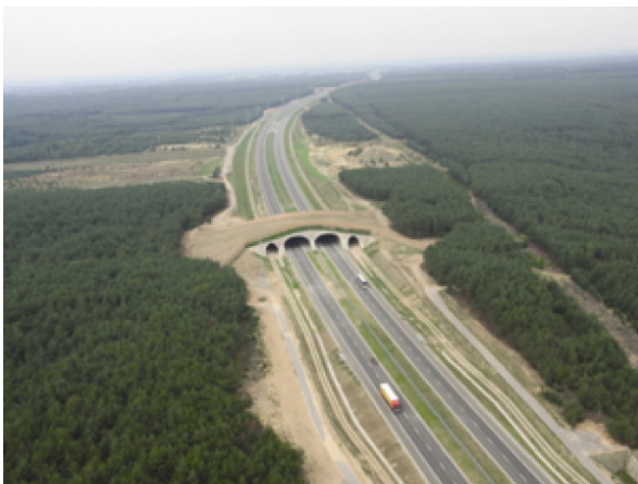
Fig. 15. An example of an overpass for animals (medium and large size) on the A1 Motorway (Poland), made from corrugated steel plate elements
