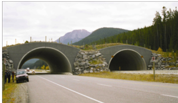
Fig. 11. An example of lack of blinding barriers on an ecobridge in Canada (Jedrzejewski 2007)
