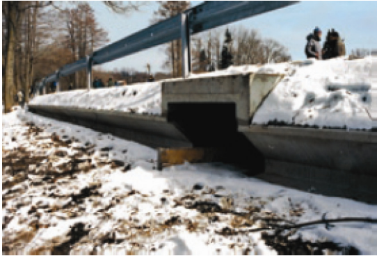
Fig. 5. Underpasses in the Czech Republic: a) for small animals (the A4 Motorway, Poland), b) for amphibians (Jedrzejewski 2007)
