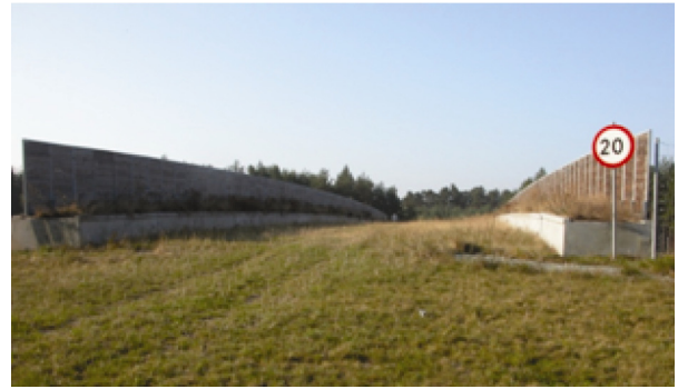
Fig. 10. A view of an animal crossing inlet – a road sign and concrete flower beds
