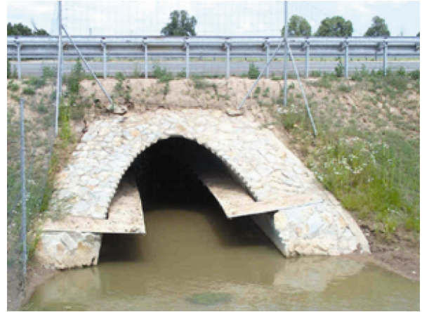
Fig. 16. An example of a typical underpass (elliptical shape) with shelves for amphibians above the high water level in Poland
