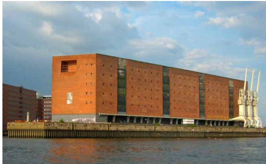
Fig. 4. Conversion example of replacing the facade while retaining the carcass (Keičiasi Miestai 2015)
