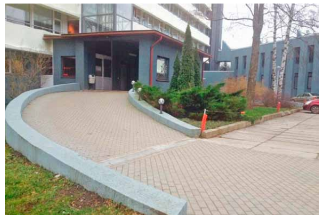
Fig. 8. The comfortable ramps for wheelchairs and prams in the rehabilitation centre Vaivari. Source: L. Balode's private archive, 2014
