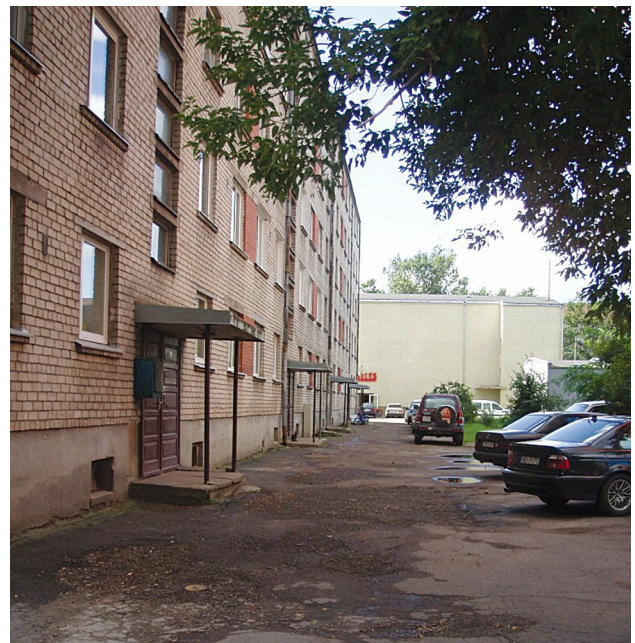
Fig. 1. Dilapidated courtyard territory, example in Latvia
